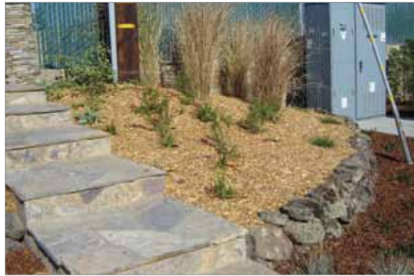
DISPLAY 19 STAIRWAY & RETAINING WALL
