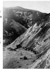
crusher. It produced 20 tons of  $2\frac{1}{2}$  inch rock per hour. The granite was transported from the quarry face in horse-drawn, side-dump rail cars, still loaded by hand.
